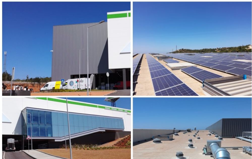
Figure 2. Front facade and roof with photovoltaic panels of the case study store in Algarve, Portugal.
