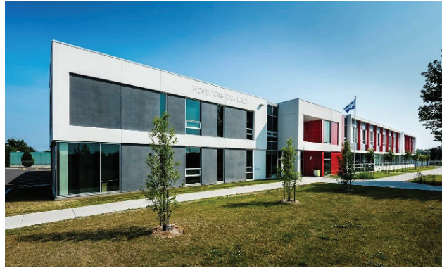
Figure 2. Electrically heated school building, Horizon-du-Lac (near Montreal, QC, Canada).
