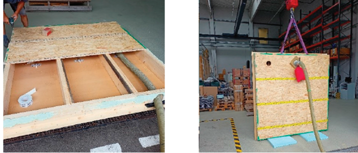
Figure 6. Horizontal position before blowing in (left) and vertical position before blowing in (right).
