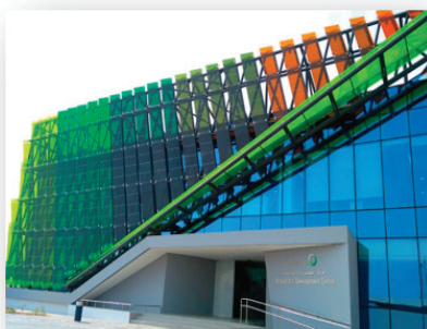
Dubai Electricity and Water Authority R&D (United Emirates) BIPV façade produce 134 kW
