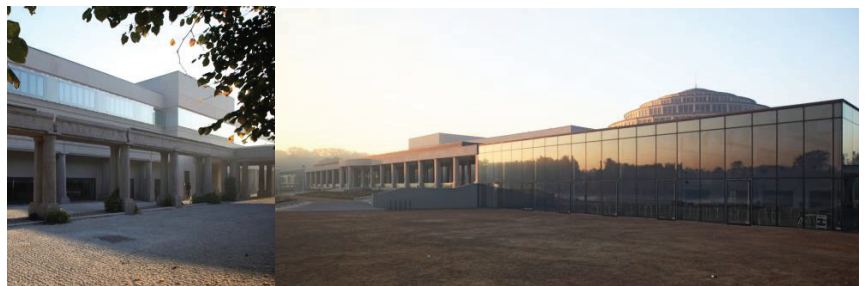
Figure 7. Renovation and refurbishment of the restaurant pavilion of the Centennial Hall complex in Wrocław—windows and glazed curtain wall (photographs by the Authors).
