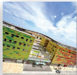
Train station (Italy) BIPV façade produce 1.0 MW
