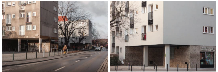
Figure 1. The blocks by Nankiera square—original and refurbished with recreated details (photography by the courtesy of Patryk Kusz/VROA Architekci).
