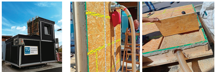
Figure 1. Outdoor test stand in Vienna (left), vertical blowing technology (middle), horizontal blowing technology (right).
