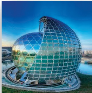
Opera Theater (France) BIPV façade produce 1.1 MW
