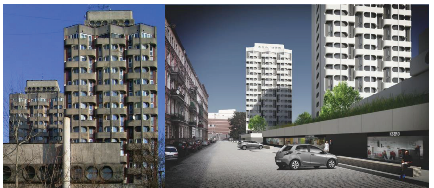
Figure 3. The renovation concept of the façades of residential buildings at Grunwaldzki square—a pre-refurbishment condition in 2007 and remodelling visualisation (photograph by the Authors).
