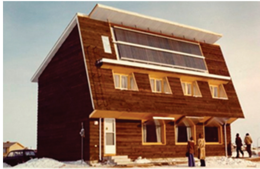
Figure 3. Saskatchewan Energy Conservation house designed by the Illinois U demonstrated passive technology in 1978 (Regina). Solar-exposed surfaces with large windows are inclined. Evacuated solar pipes are placed on the attic level. It was provided with an air-sourced heat pump and polyethylene-based heat recovery ventilator. Reprinted with the permission of Harold Orr.
