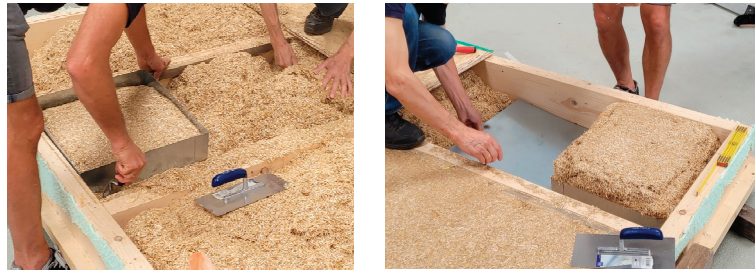
Figure 4. Sampling by means of sheet metal frame.
