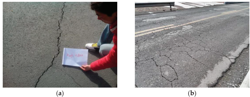
Figure 3. Lateral cracking and network cracking problems of asphalt pavement. (a) is transverse crack; (b) is net crack.
