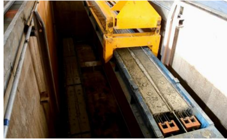
Figure 22. Steam curing of the concrete sleeper.
