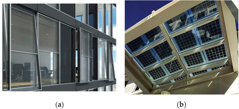
Figure 9. (a) BIPV façades powered by electricity to assist natural ventilation [186]; (b) an entrance with a PV skylight [187].
