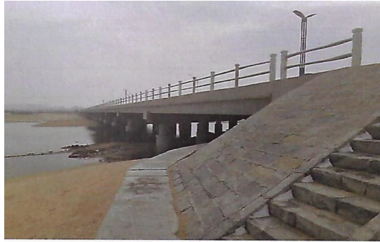
Figure 2. Photograph of the project.
