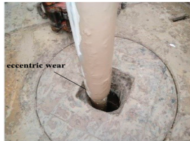
Figure 2. Off-center drill string on site.
