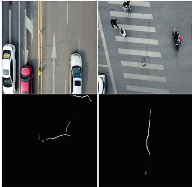
Figure 5. Segmentation of fine cracks.
