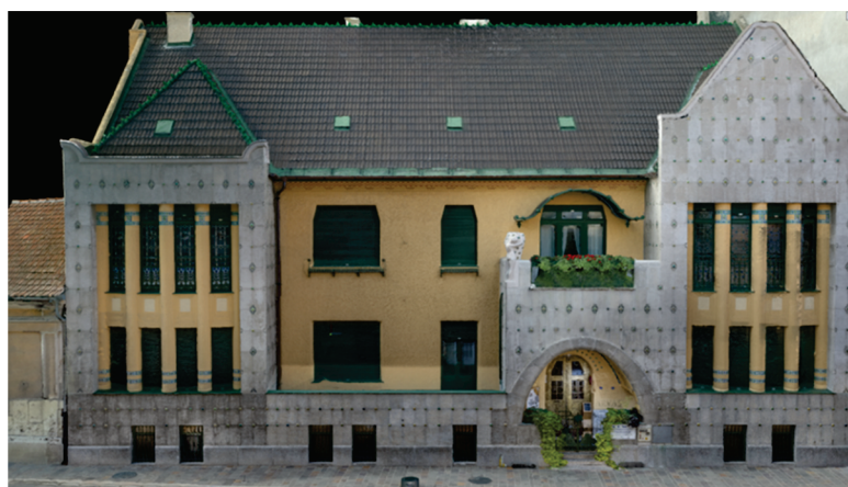
Figure 2. The main facade of Darvas-La Roche Museum House.
