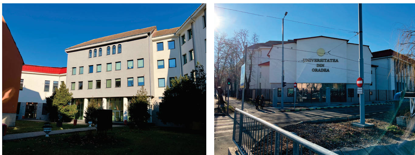
Figure 1. (a) Building F—inner courtyard façade. (b) Building F—University Street façade.
