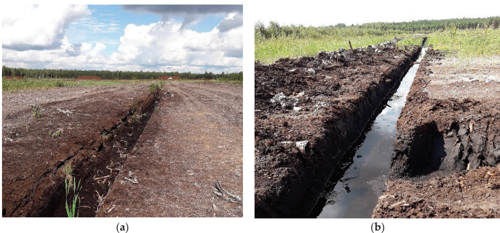
Figure 1. Drainage ditch in the study site: (a) drainage ditch before cleaning; (b) drainage ditch after cleaning.
