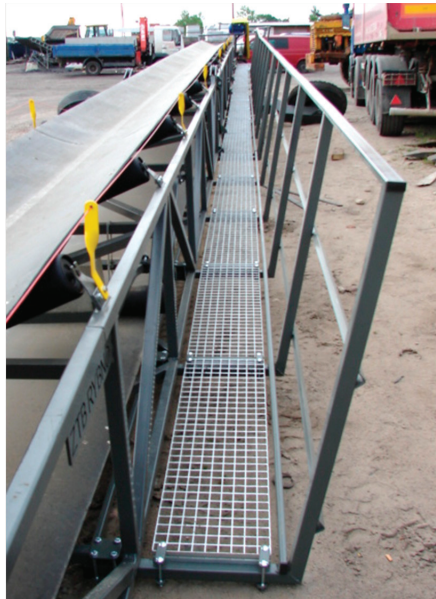
Figure 6. Belt feeder's route with a platform for the crew.
