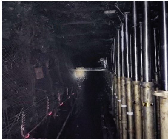
Figure 18. Effect of gob-side entry retaining.
