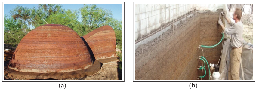
Figure 3. Ferrock construction examples. (a) Dome structure made of ferrock in USA. Picture taken from https://www.certifiedenergy.com (accessed on 15 October 2023). (b) The process of building a ferrock wall. Picture taken from https://www.pbs.org (accessed on 15 October 2023).
