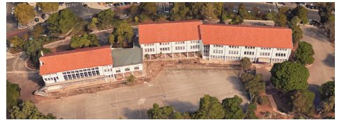
Escola Básica Paula Vicente 3 × 3 reinforced concrete pavilion (“3 × 3”)
