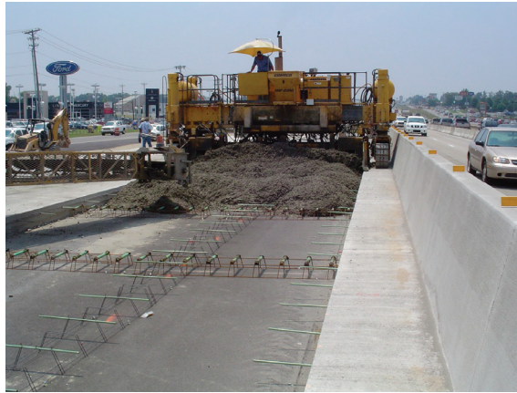
Figure 1. Typical legacy concrete pavement repair in progress.
