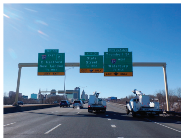
Figure 1. Sign support 21311 on I-84, Hartford, CT.
