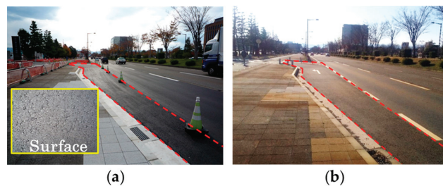
Figure 4. Views of the test section in Ishikawa Prefecture ((a) 2019 and (b) 2021).
