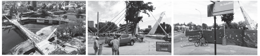
Figure 16. (left to right) Road disruption during construction: the main source of negative reporting, affecting pedestrian and bicycle traffic as well as key trunk services for almost two years. (Credit: Left: From public television broadcast (Cordoba Governance); Centre and Right: reproduced with permission from the author Mr. Mario Rojas (Centenario digital publication)).
