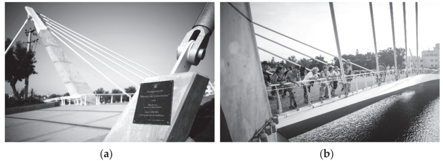
Figure 13. (a) Exposed stay attachments as ‘honest’ engineering themes. (b) Various activities were observed in the wider areas of the deck, without interfering with the central pedestrian flow.
