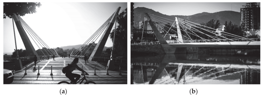
Figure 14. (a) Masts raising upwards and outwards resemble welcoming ‘open arms’. (b) Masts, abutment walls, and foundations form an integral element.
