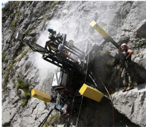
Figure 32. Roboclimber field deployment “Reprinted/adapted with permission from Molfino et al. [151], Elsevier”.
