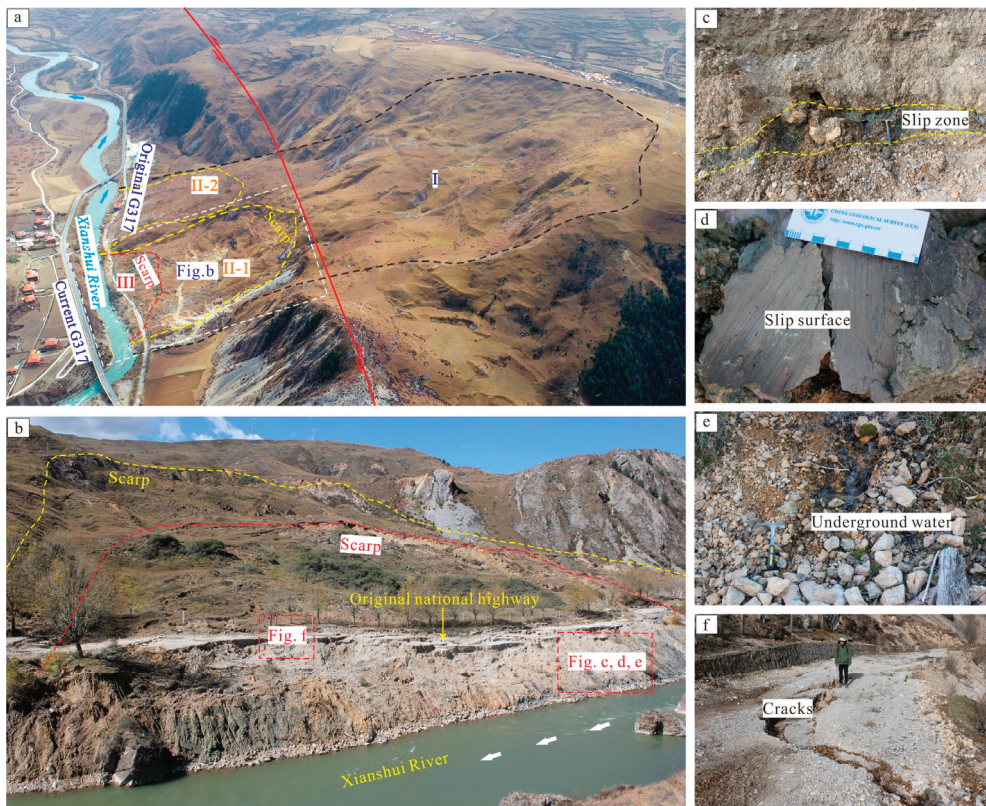
Figure 7. Reactivation features of the Dandu landslide: (a) overall view of the Dandu landslide; (b) deformation zone at the front of the landslide; (c) slip zone at the landslide's toe; (d) slickensides on the slip surface; (e) groundwater outflow along the slip zone; and (f) cracks in the front of the landslide.
