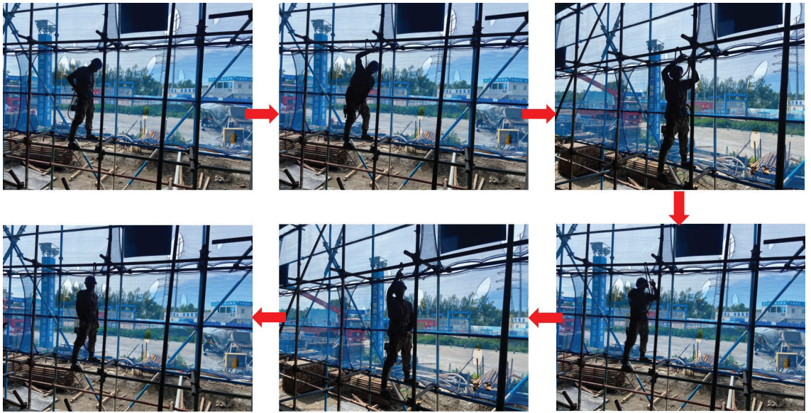
Figure 2. Field test of safety rope fastening.
