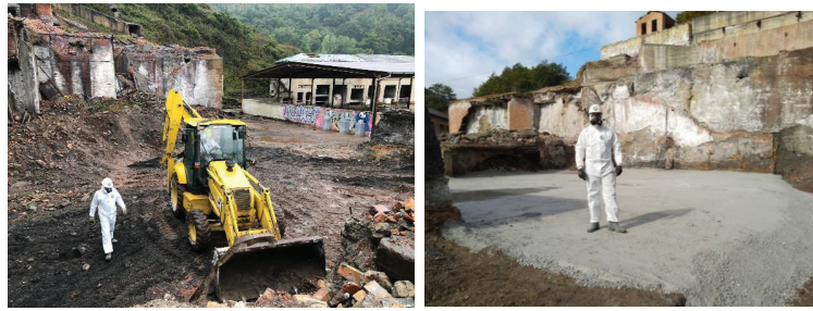
Figure 10. (Left): task 1 (debris removal); (Right): task 2 (concrete slab construction).
