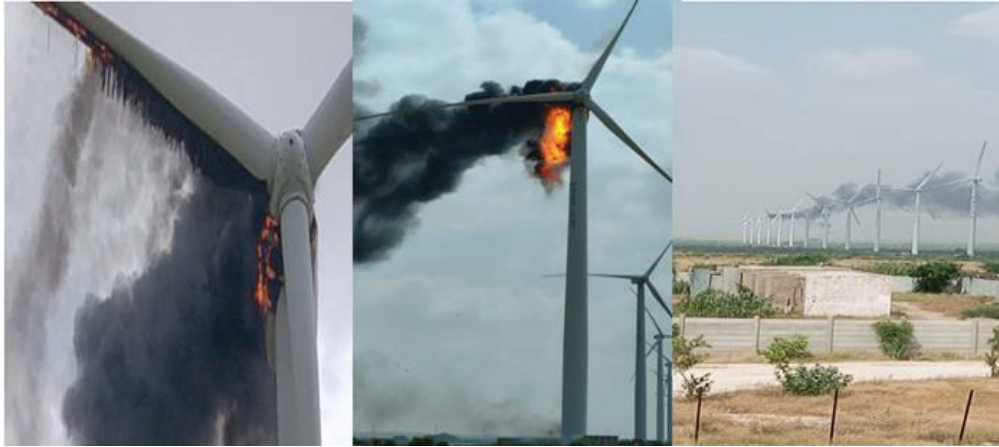
Figure 3. Extend of damage due to wind turbine failure during October 2022 at Sapphire Wind Power Plant at Jhimpir.
