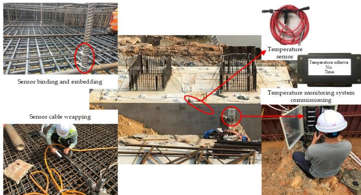
Figure 2. The temperature monitoring system of mass concrete in this study.
