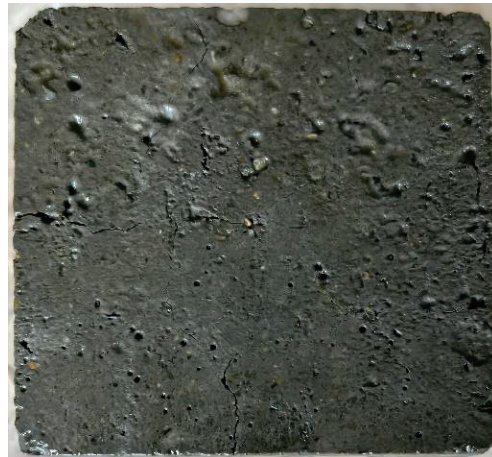
Figure 1. Surface of concrete specimen after pretreatment.
