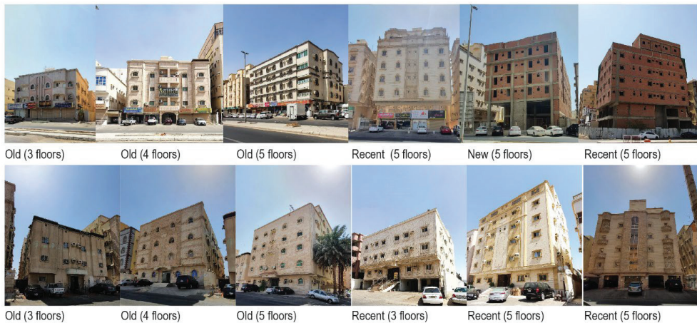
Figure 7. Different types of low-rise residential buildings illustrate the types of construction and ownership.
