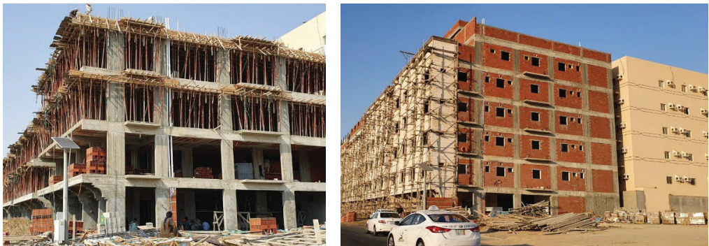
Figure 9. The 20 cm blocks for wall-filling within the skeleton structure.
