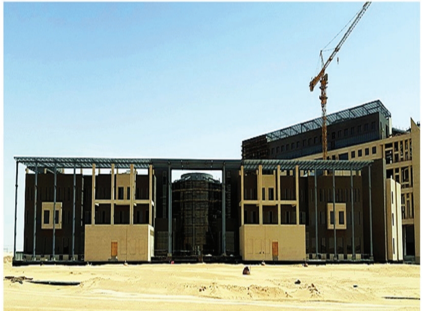
Figure 4. Outpatient ward façade.
