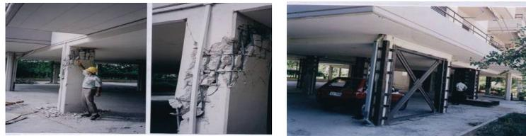
**Figure 3.** Damaged columns at the soft-story and temporary steel shoring.
