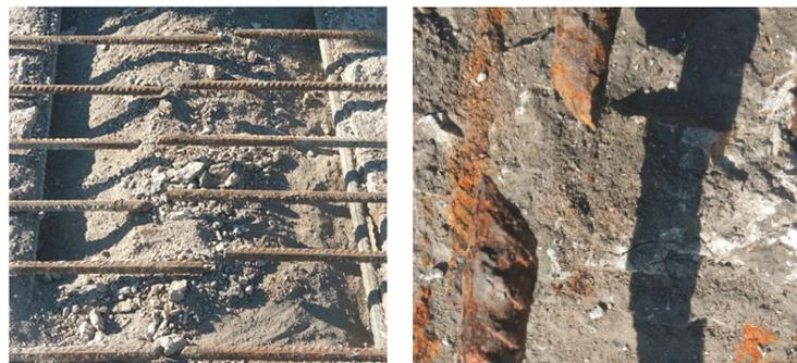
**Figure 7.** Sectional cuts in the transverse reinforcement bars.
