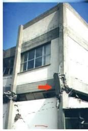
**Figure 4.** Damaged short columns from the interaction of unreinforced masonry infills (UMI), built within the bay of an RC frame structure, with the adjacent RC columns.
