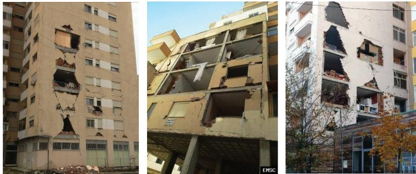
**Figure 9.** Out-of-plane collapse of unreinforced masonry infills (UMI) panles from RC frame structures due to earthquake excitation.
