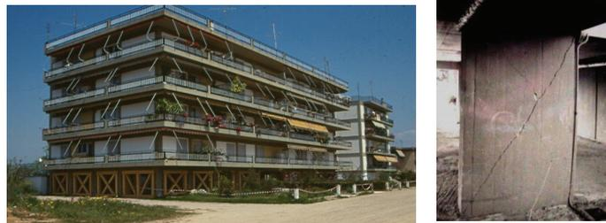
**Figure 2.** Temporary wooden story. Damaged shear wall at the soft story.
