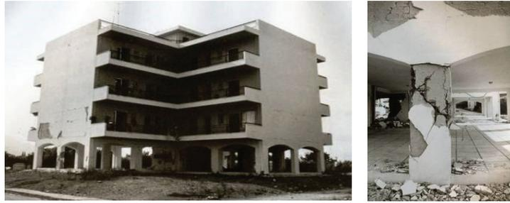
**Figure 1.** Damaged columns at the soft story.
