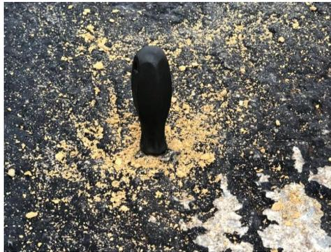
**Figure 8.** Venting pipes check to verify the clogged conditions (see the handle of the screwdriver inserted into the hole).
