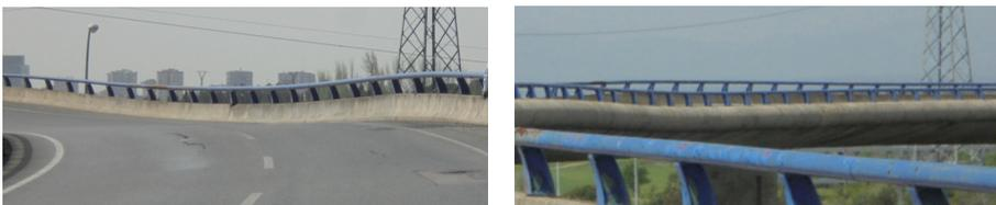
**Figure 4.** Marked deflections in spans # 5 and # 8 of Nudo de Colmenar structure.
