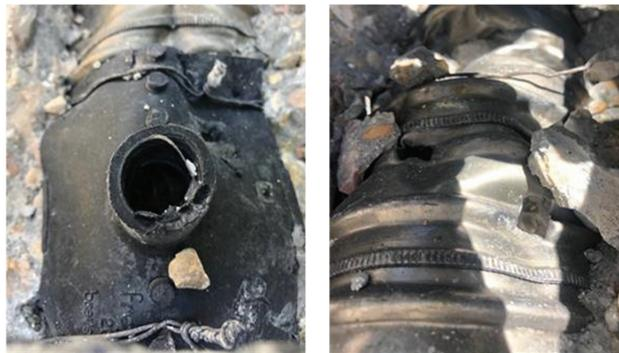
**Figure 11.** Lack of connection between venting pipe and prestressing sheath (Colmenar Bridge).
