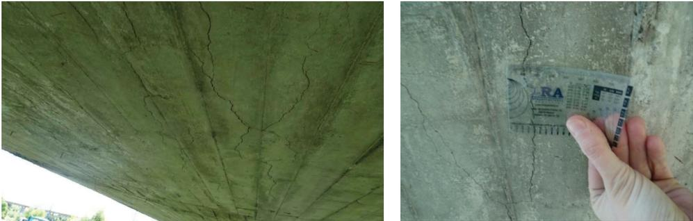
**Figure 3.** Longitudinal cracking on the bottom surface of the deck.
