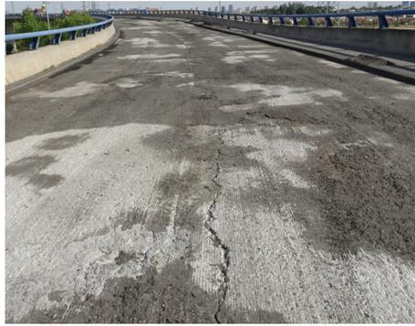
**Figure 5.** Longitudinal cracks in the deck's upper face.
