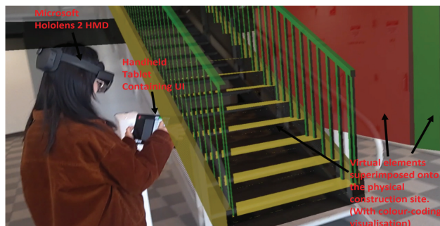
Figure 2. This figure shows a third-person perspective of the BIM-ARDM system. The BIM model is superimposed over the physical site at a one-to-one mapping. A colour-coded visualisation represents correct (green), minor (yellow), and major (red) defects.
