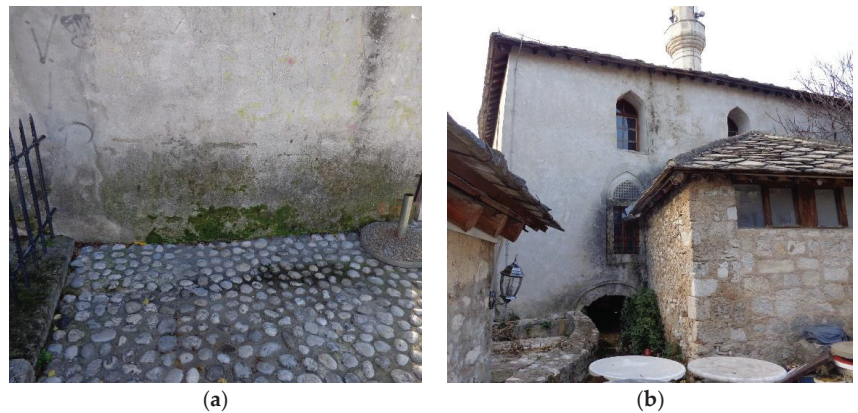
Figure 4. (a) Ascending moisture and biological attack (author's photo, 2023). (b) Descending moisture (author's photo, 2023).
