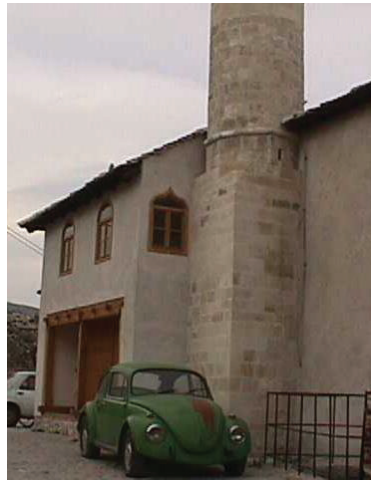
Figure 7. Vertical joint between the minaret and the mosque building, no plaster spalling visible shortly after reconstruction (author's photo, 2020).
