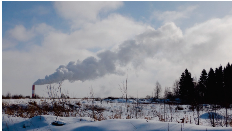
Figure 12. The view of the Petrozavodsk thermal power plant (the Republic of Karelia).
