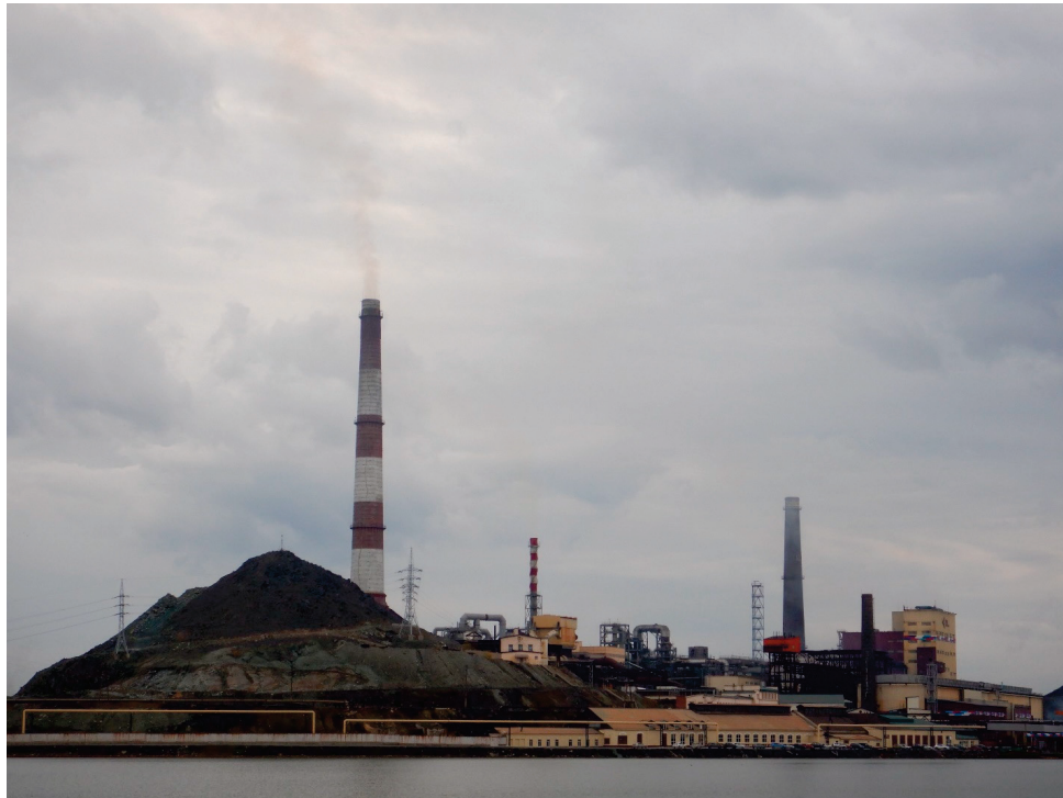
Figure 2. The view of Karabashskiy Copper-Smelting Plant (photo by the author).
