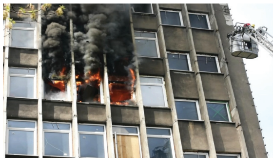
Figure 7. Windows breaking during the second test fire.
