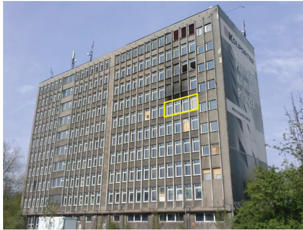
Figure 1. View of the building with the test room marked (on the west façade).
