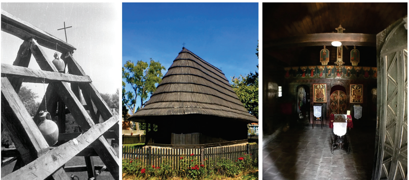
Figure 3. Wooden church in Brzan village: acoustic vessels hanging on the roof construction as found during the reconstruction works in the 1960s ( left ), church exterior ( middle ), church interior ( right ) (photo: Institute for the Protection of Cultural Monuments of Serbia ( left ), Zorana Đorđević ( middle and right )).
