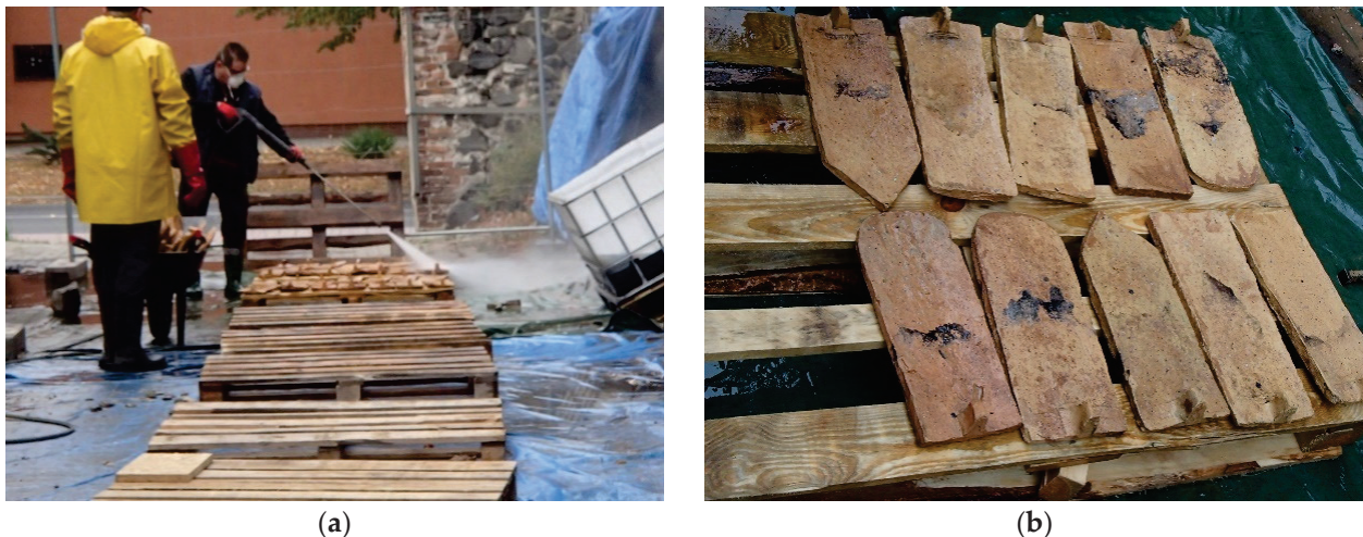
Figure 3. Revitalization of historic roof tiles: (a) cleaning; (b) maintenance.
