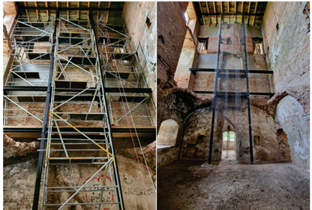
Figure 14. Current view of the strengthened wall and the strengthening structure (photos by authors).
