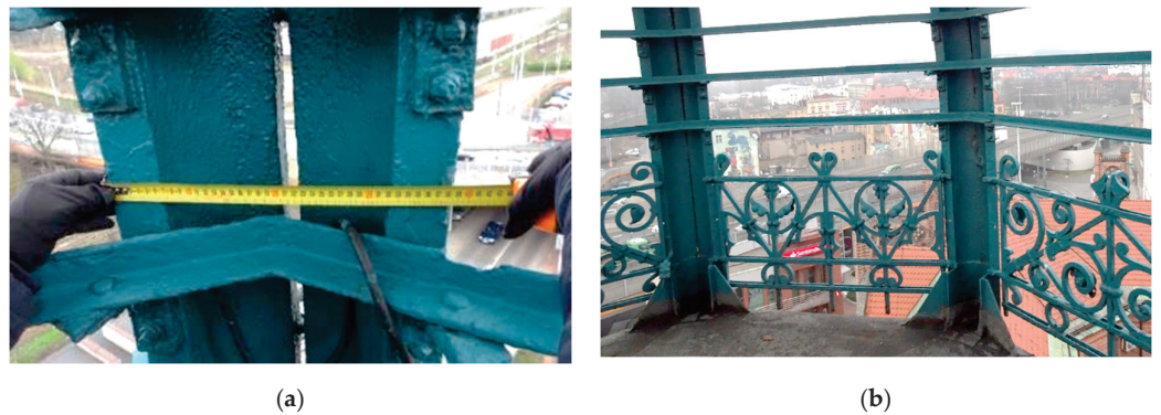
Figure 4. Steel dome structure. (a) View of the balustrade surrounding the dome; (b) the 38 cm width of one of the dome's eight supporting ribs.
