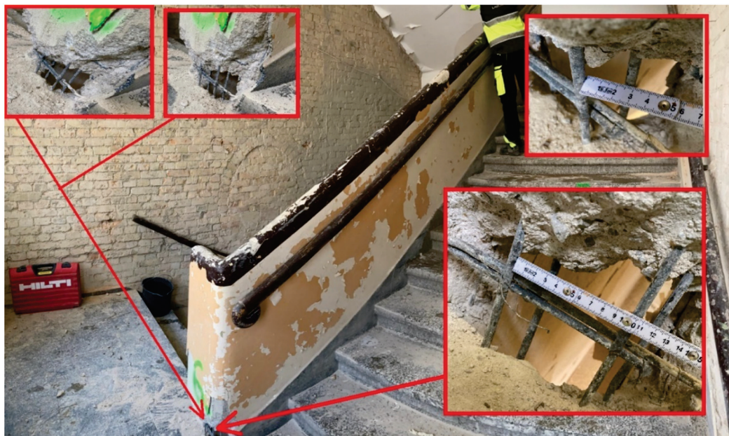
Figure 3. A view of a staircase with a sample 8 location.
