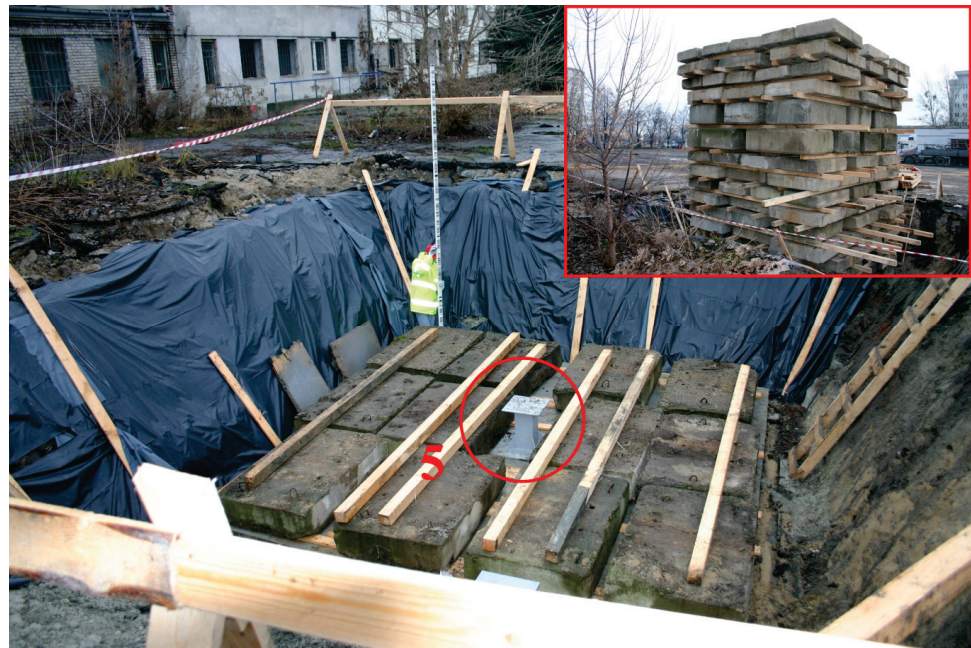
Figure 3. Positioning of benchmark no. 5 and concrete plates view.
