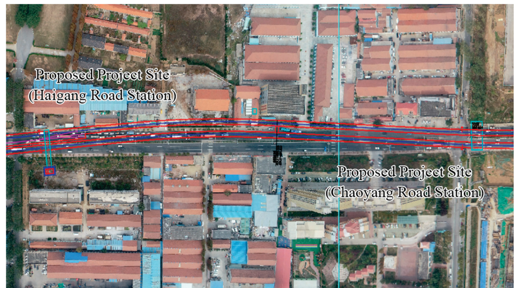
Figure 3. Aerial photo of the proposed tunnel construction section between Haigang Road Station and Chaoyang Road Station.
