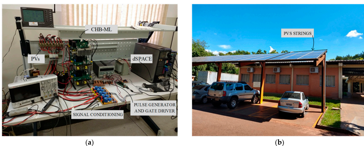
Figure 8. (a) Experimental setup for the seven levels cascaded H-bridge inverter; (b) Photovoltaic panels: Sun Earth PV-Module 235 W.
