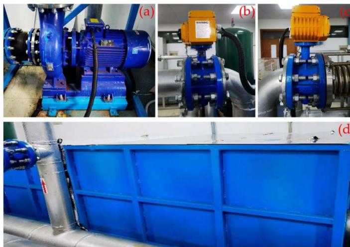
**Figure 3.** Physical pictures of the water supply module device: (a) QZHW200-250IA centrifugal pump; (b) motorized butterfly valve; (c) motorized regulating valve; (d) low-level water tank.
