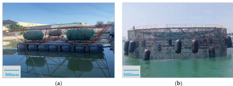
Figure 1. Steel grid structure with bolted ball joints: (a) Floating platform; (b) Deep-sea fish cage.
