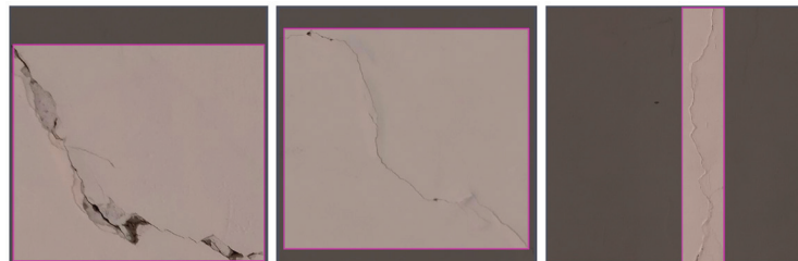
Figure 2. Annotated images in the dataset. Bounding box for cracks detection.
