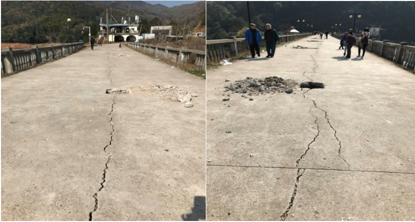
Figure 1. Dam crest of Wujing reservoir.
