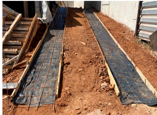
Figure 4. Application of tarp on the ramp floor before concreting.
