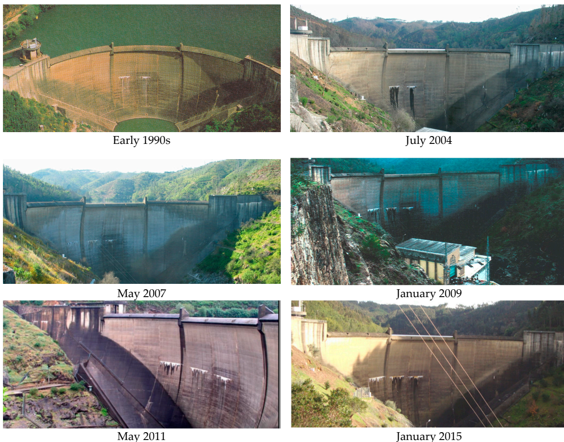
Figure 5. Downstream surface appearance from early 1990s to January 2015.
