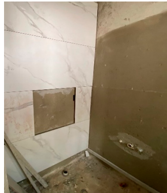
Figure 6. Bathroom after applying waterproofing.
