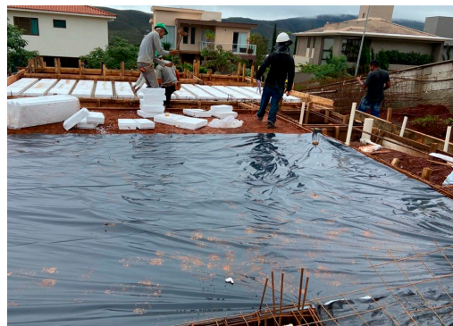
Figure 2. Application of tarp on the floor before the concreting.
