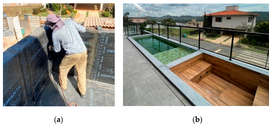
Figure 10. (a) Application of chicken wire over pool blanket; and (b) pool, fireplace, and deck.
