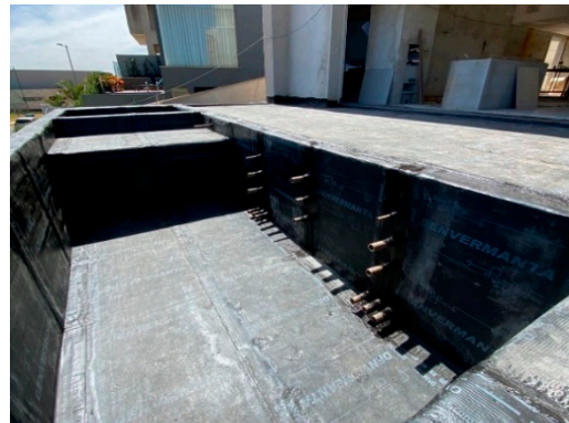
Figure 8. Swimming pool with polyethylene asphalt blanket applied.
