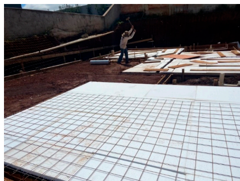
Figure 3. Positioning of EPS plates.
