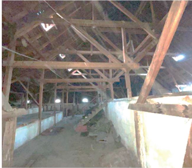
Figure 5. Image displaying the uninsulated attic.
