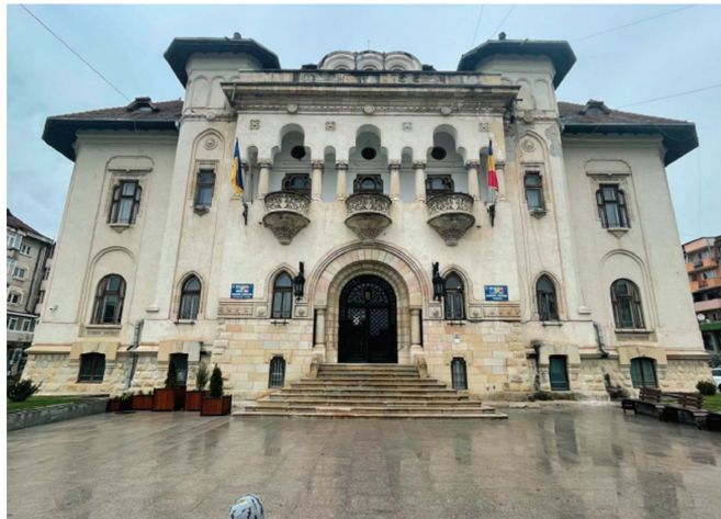
Figure 2. Town Hall of Câmpulung, Romania—main façade, showcasing the neo-Romanian style.
