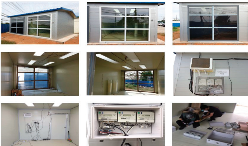
Figure 9. Construction of test and reference rooms.
