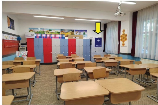
Figure 3. Photo with the second heat recovery ventilation unit placed in the school.
