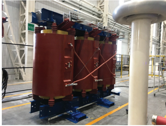
Figure 24. Actual arrangement of transformer voltage test.
