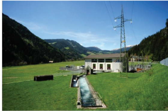
Figure 2. Hydroelectric power plant.
