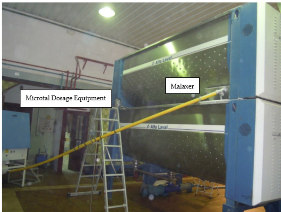
Figure 2. Malaxer and NMT dosage equipment at the ‘Aceites San Antonio S.L.U.’ olive mill.
