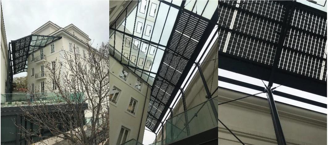
**Figure 7.** Positive example of the “*reversibility*” criteria on the solar intervention of Palazzo Leonori in Rome (Italy), where the transparent BIPV roof is detached from the original XIX Century Palace by metallic columns [75] (Source: Elena Lucchi).
