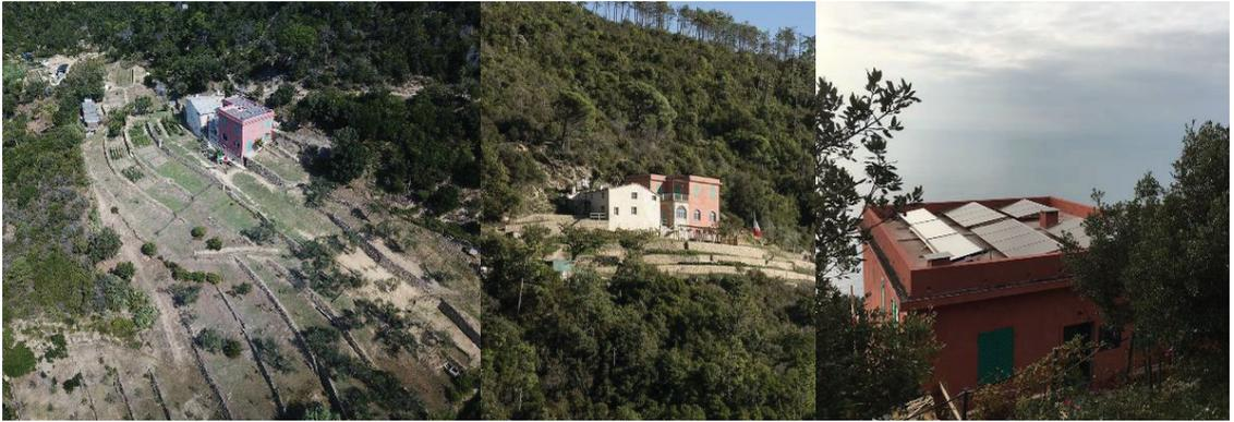
**Figure 10.** Positive example of the “concealment” of the solar intervention in the Podere Case Lovara in Levanto (Italy) thanks to the presence of traditional PV and ST panels hidden behind a parapet and not visible from the protected landscape of the Cinque Terre Natural Park (Source: Fondo per l’Ambiente Italiano).
