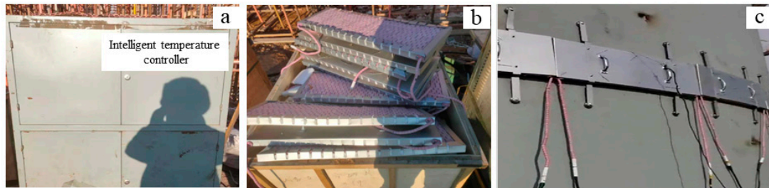
Figure 1. Ceramic heating-related device. (a) Temperature control box, (b) ceramic heating plate, and (c) ceramic heating construction.
