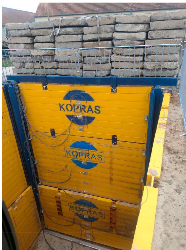
Figure 5. Loading of the backfill with 10 layers of road slabs ( 38.4 \text{ kN}\cdot\text{m}^{-2} ).
