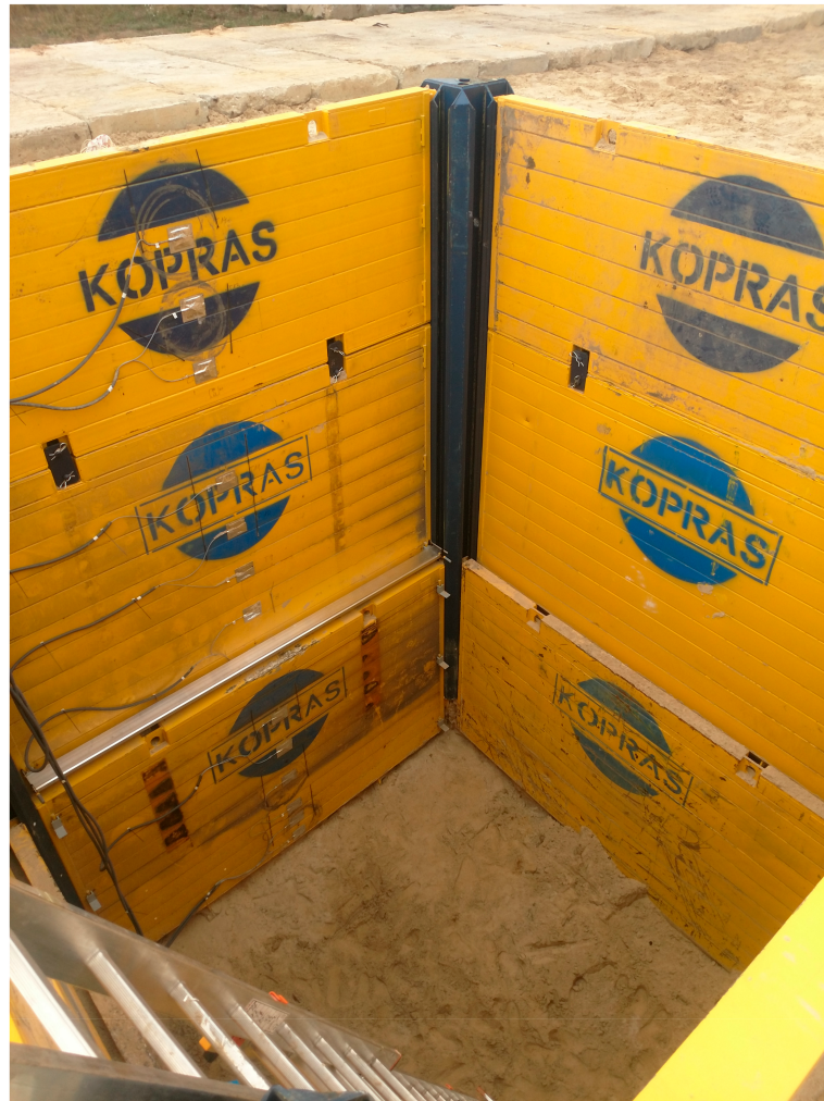
Figure 2. Test stand—view of the excavation and the excavation support.
