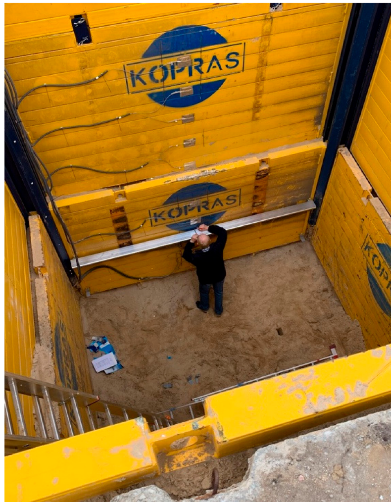
Figure 6. Direct measurement of the deflection arrow taken with a measurement patch.
