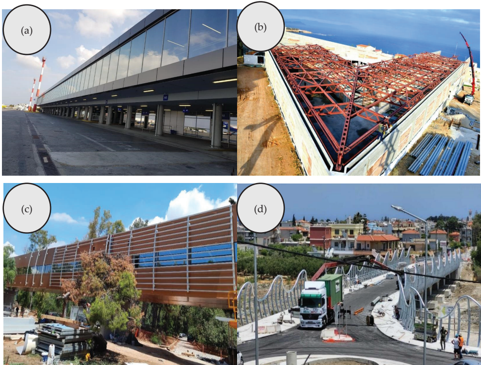
Figure 1. (a) Airport, (b) roof canopy, (c) pedestrian bridge, (d) bridge railing.
