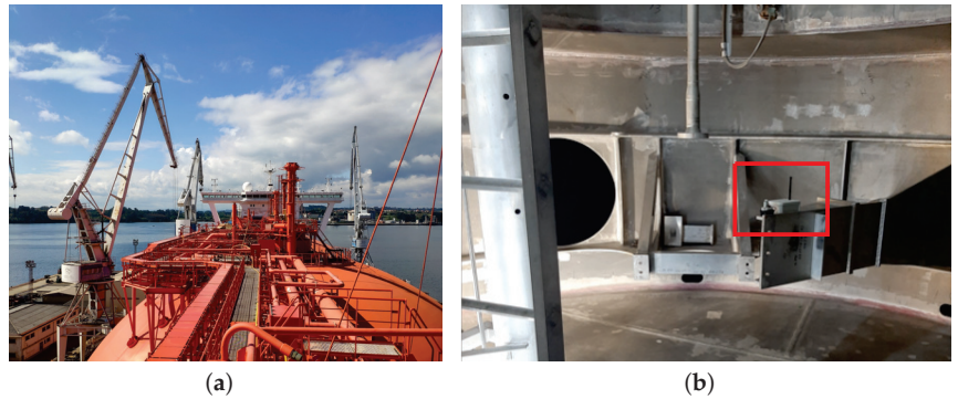
Figure 4. Gas carrier where the system was tested (a) and ORP IoT device placed inside a tank of the gas carrier (b).
