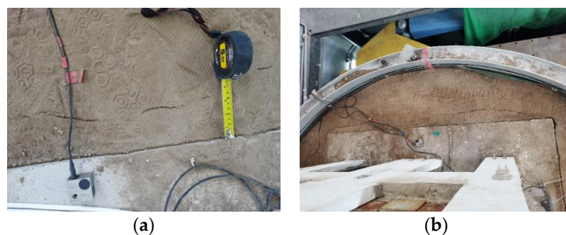
Figure 6. Cracks on surface of soil around the foundations after 0.20 g seismic motion input. (a) Test of pile group foundation model. (b) Test of raft foundation model.
