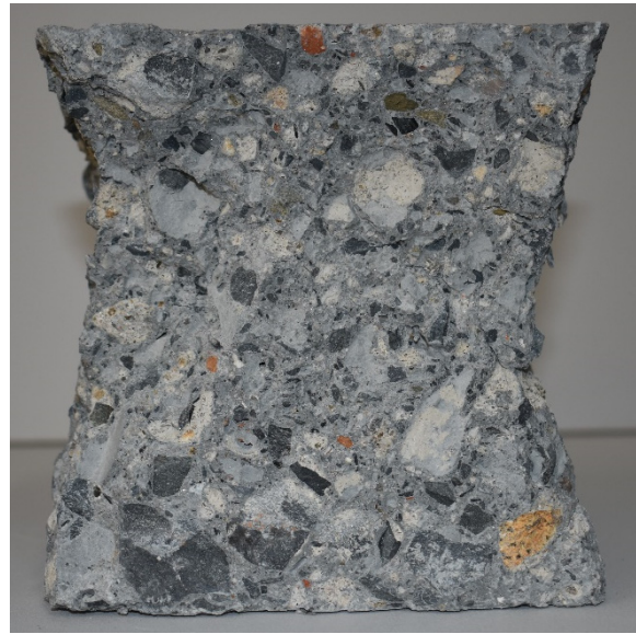
Figure 10. Failure mode in HR-100+50 mix.
