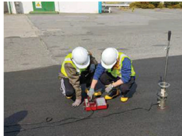
Figure 8. On-site Light Falling Weight Deflectometer.
