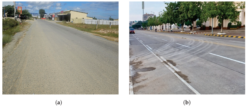
Figure 15. (a) MAST pavement and (b) concrete pavement where the pass-by tests were conducted.
