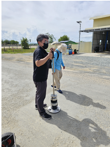
Figure 7. LFWD testing device.
