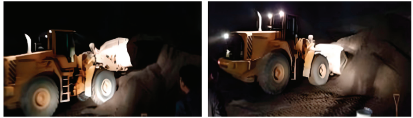
Figure 2. Collecting of RAP aggregate in the asphalt plant.
