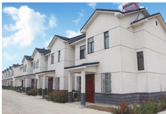
Figure 2. Buildings with CFS-CLPM composite walls.
