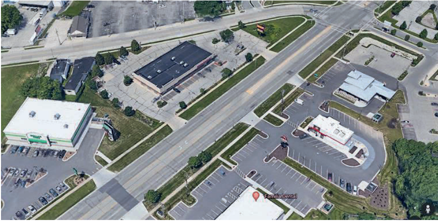
Figure 4. Reversible “suicide” lane with yellow lane markings as the centermost lane of US Highway 141. Source: Google Maps (2021e)—Reversible Lane, @ 44.49, -87.97.
