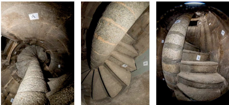
Figure 6. Fisheye views of the internal winding of the staircase.
