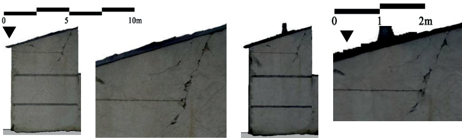
Figure 17. Orthoimage of the East side. The aerial model by integrated oblique and nadir cameras (right), can be comparable in terms of available detail and the accessible information to the terrestrial photogrammetric one (left).
